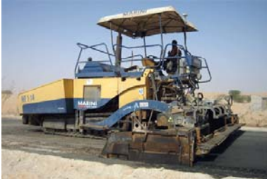
Finisher (Asfalt Serme)
